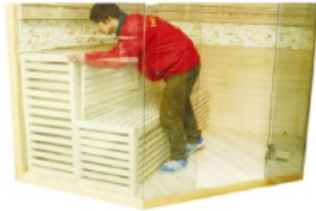
FIG-15 Assembling sitting board's support
