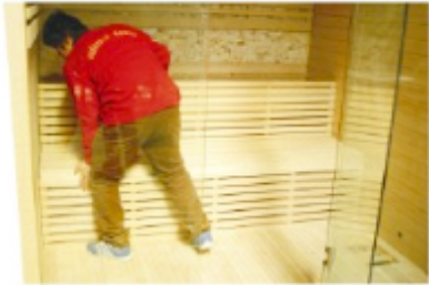
FIG-14 Assembling sitting board's support
