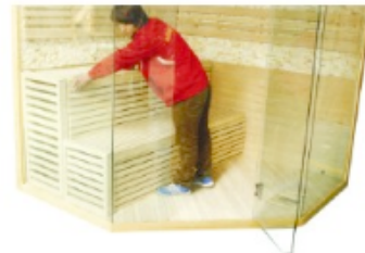
FIG-16 Assembling sitting board
