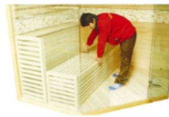
FIG-14 Assembling sitting board
