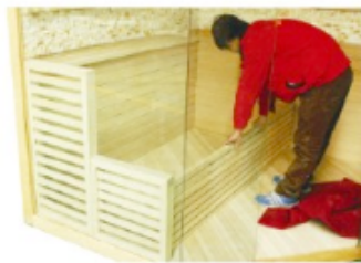
FIG-13 Assembling sitting board's support
